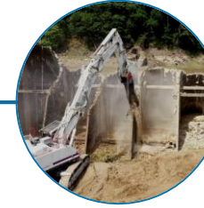
2022 Removal of LRQB dam
