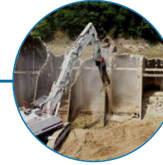
2022 Removal of LRQB dam
