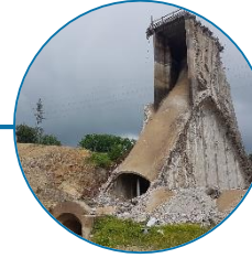
2020 Removal of Vezins dam
