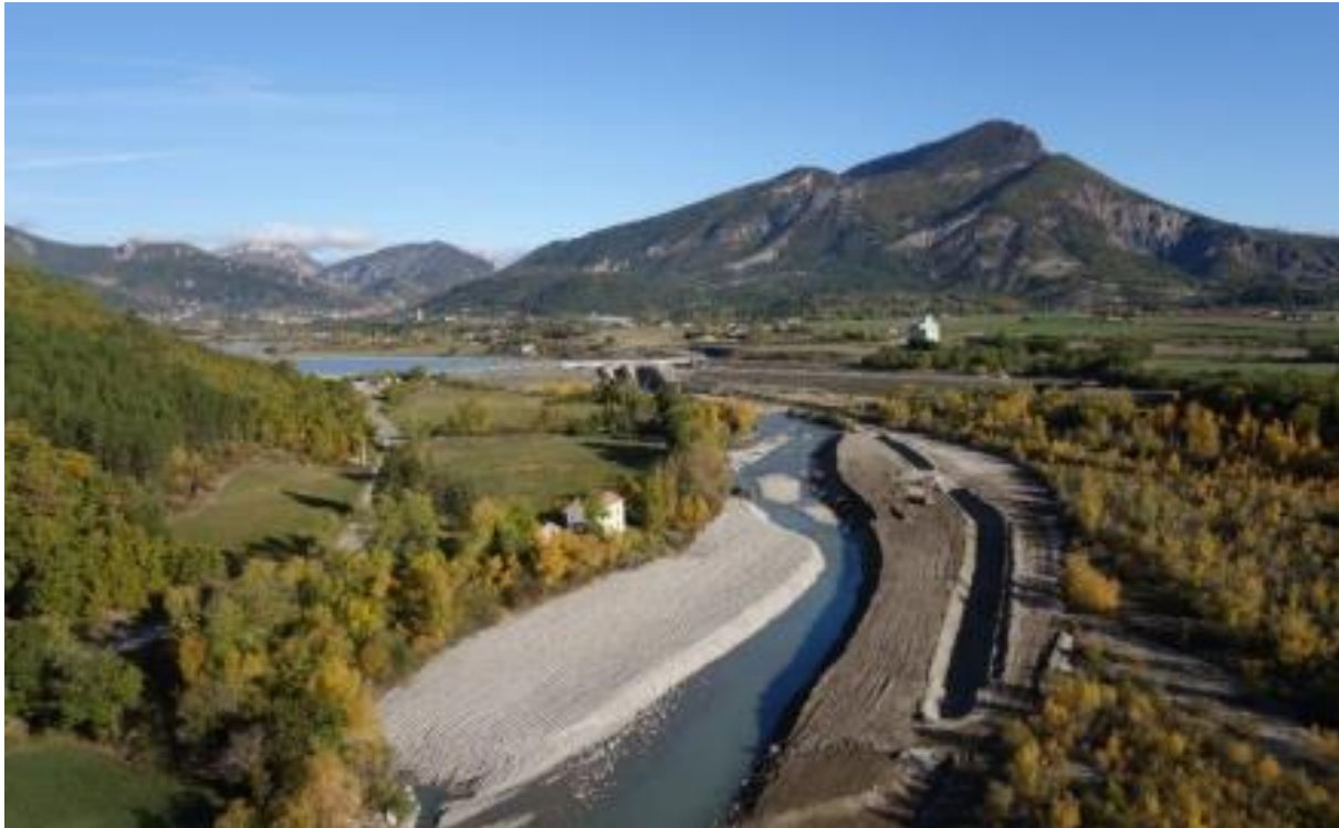
Reinjection of sediment downstream of the St sauveur dam
