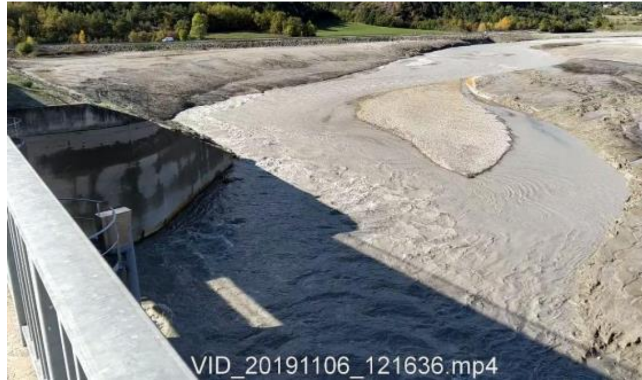
Opening of St Sauveur gates during a flood to let sediment pass (EDF)
