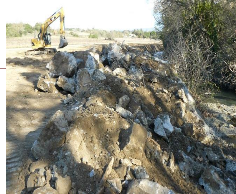
Destruction of bank protections and walls (SMMAR)
