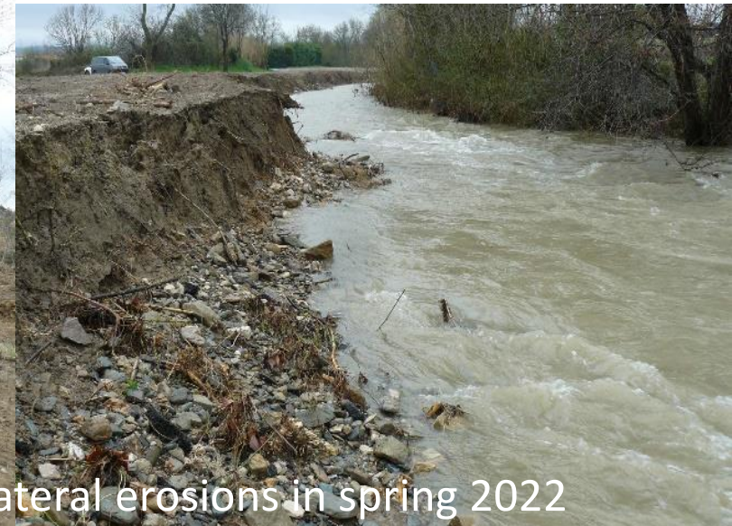
Destruction of bank protections and walls (SMMAR)
