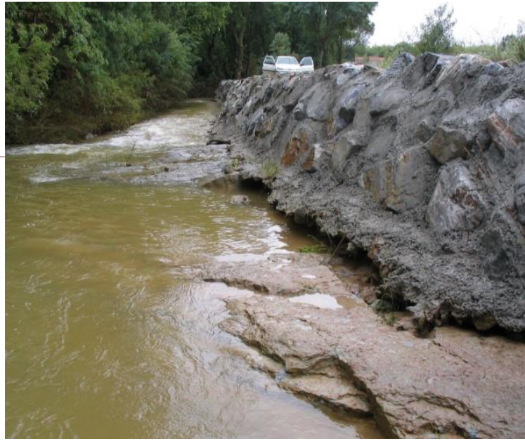
The Clamoux river, along the RD 37 road before work. The river is constrained, it incised and bank protection is needed after each flood
