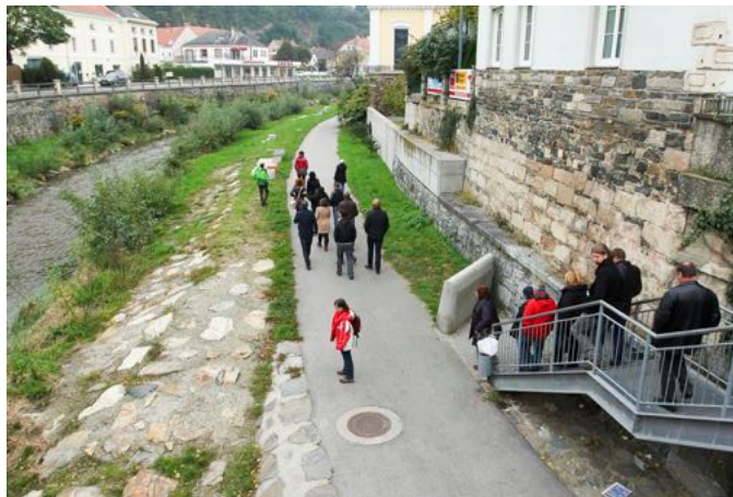
A restored section of river Krems was visited on one of the excursions of the 6th ERRC. The footpaths allow people to come close to the river and enjoy it, while the flood barriers make sure area surrounding the river stays dry during the regularly occurring flash floods.
