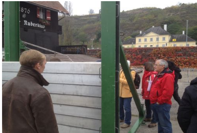
The mobile flood barriers along the Danube were visited in one of the excursions of the 6th ERRC. These provide protection against high water events, while allowing contact between the town of Stein and the river.
