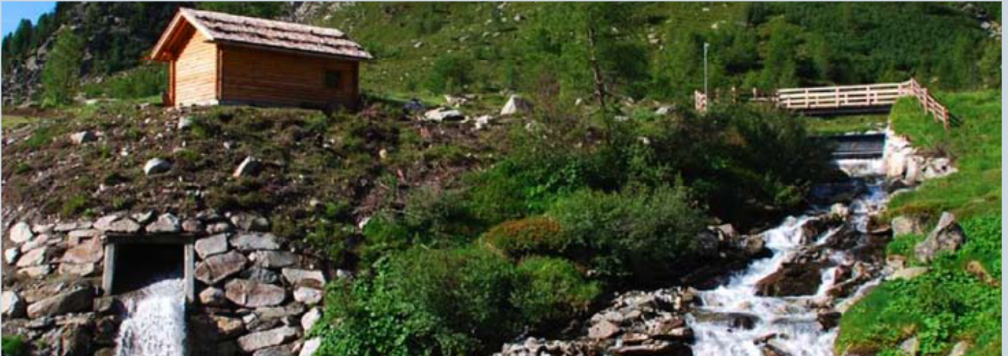
Panoramic view of the inlet structure
