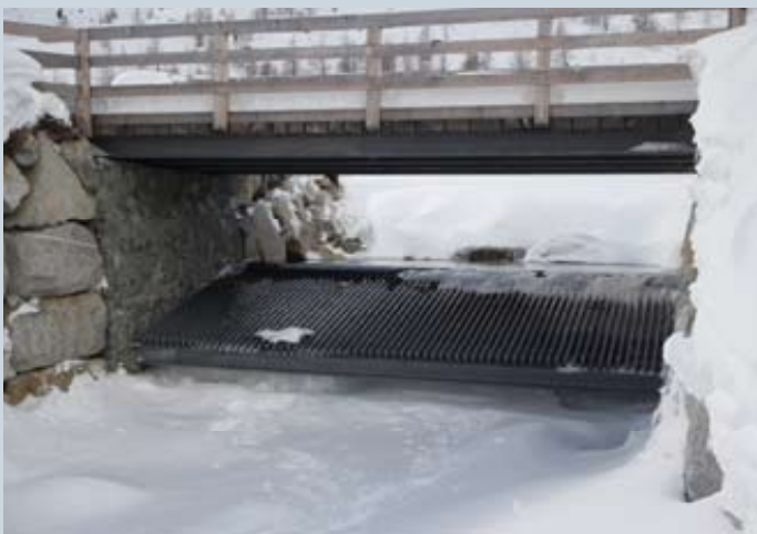
Detail of the inlet structure
