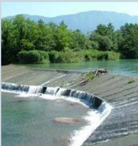
Dam for HPP Gradišče on the river Vipava
