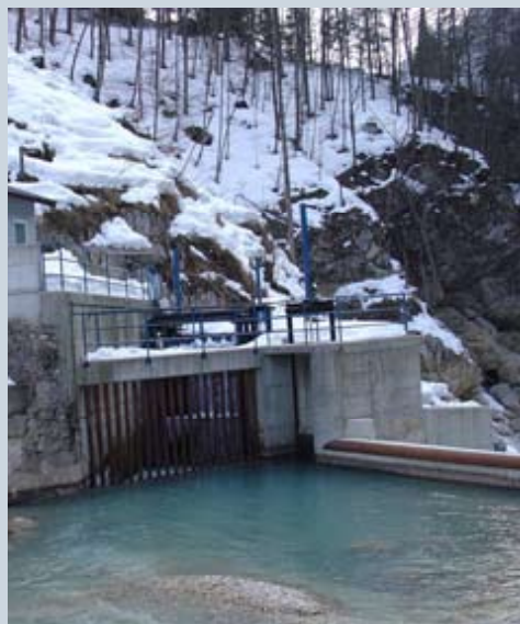
Intake structures of HPP Možnica on the river Koritnica
